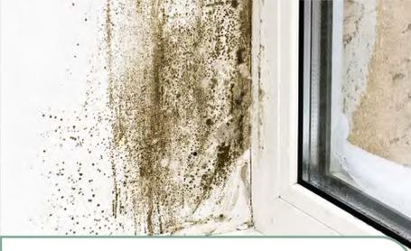
***Where condensation is the cause of mould there are no repairs to cure it. The only way to cure it is by following the advice in this leaflet.***
